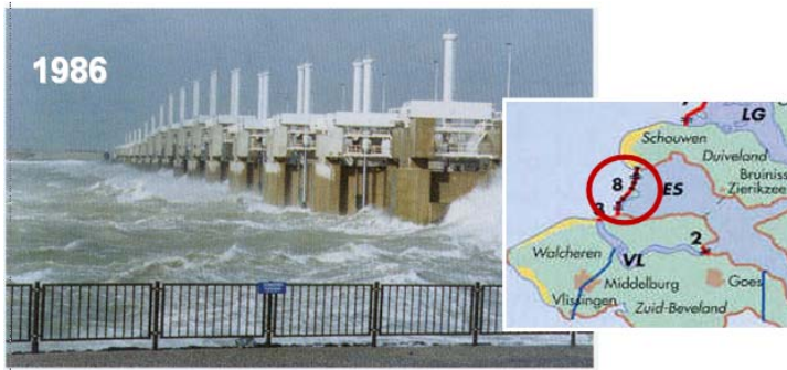
Figure 3.C.2 : Movable sea defense system along the Dutch coast. Delta works, Zeeland (RWS 2009)
